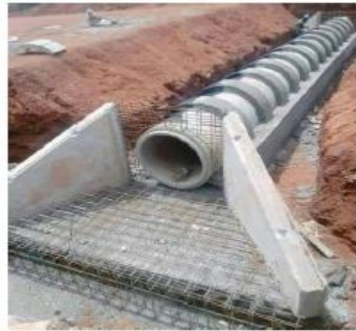
Gambar IV.9 Cross section Drainase Cross section tol Cikampek
